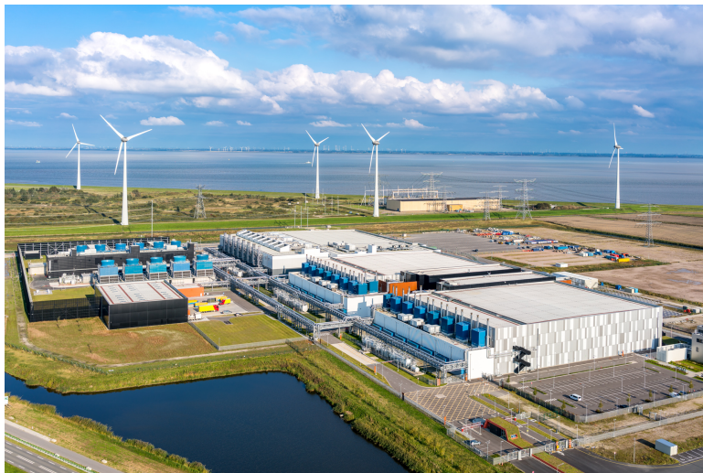
Figure: Google data center in Eemshaven, Netherlands ( google.com/about/datacenters/ )
